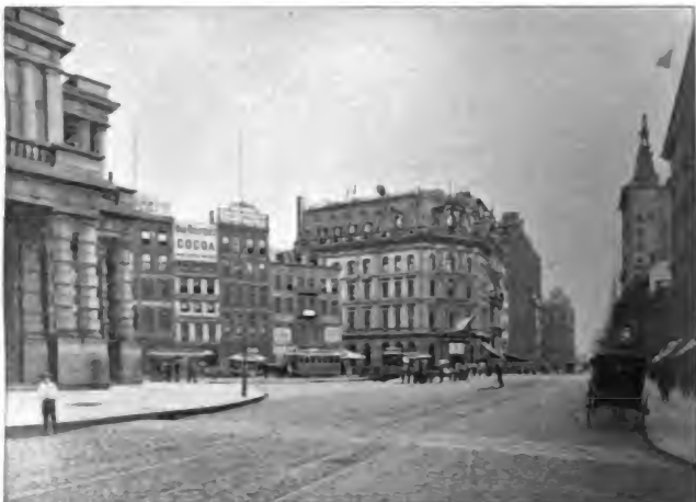
NEW-YORK HERALD BUILDING, BROADWAY AND ANN STREET.
